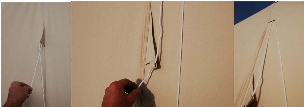
Take the end of a guy rope with an adjuster and thread it through the top loop top to bottom. Then pull it down and through the second loop (top to bottom). Make sure you thread through the end without the adjuster.
