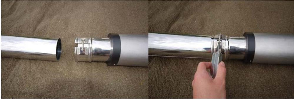
Take a clamp and screw the two parts together
